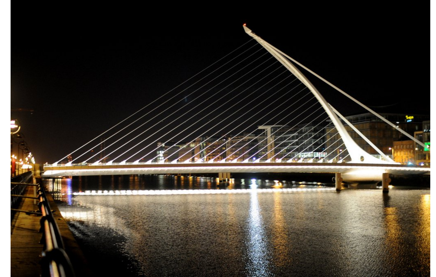
The Samuel Beckett Bridge in Dublin which drew inspiration for the bridge being presented.
